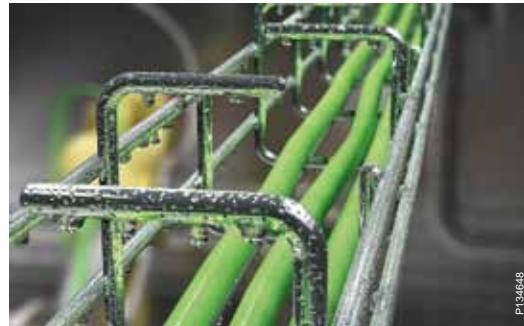
You can let loose the high-pressure washing system with no worries. Defem mesh trays withstand the most rigid sanitary regulations and the non-bundled cables will stay in place during cleaning.
